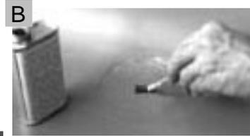
3 Roughen the penciled-in area with medium sandpaper (see fig. A). Tie-Down D-Rings are pre-roughened for your convenience. Don't risk cutting the threads under the pad, roughen only the boat.
